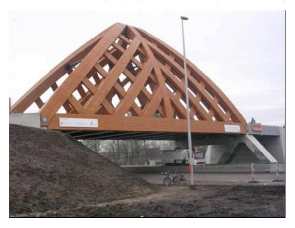
The lumber was subsequently acetylated (chemically modified) by Titanwood in Arnhem, Netherlands, to make it stable and durable for use in the bridge project. This acetylated lumber goes by the tradename - Accoya®. It was then laminated in Germany and formed into the various bridge components.
